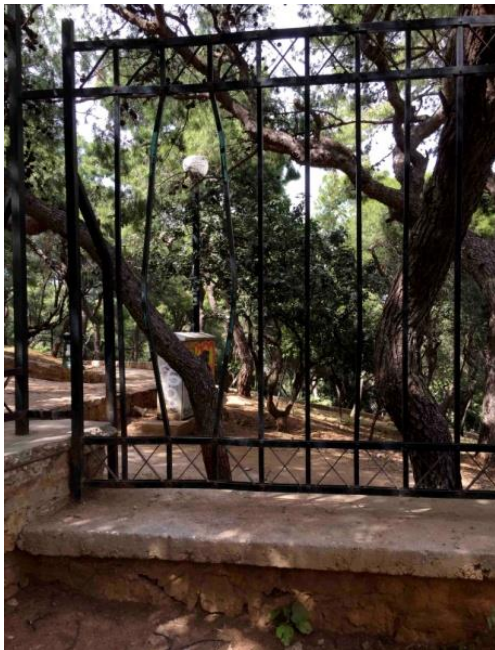
Figure 3. In order to keep up with their daily training athletes access the hill through an opening in the fence. Photo by the author and T.P., May 2020.
