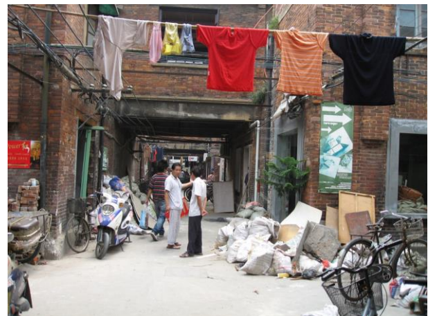
Figure 5b. During renovation (photo by the author)
