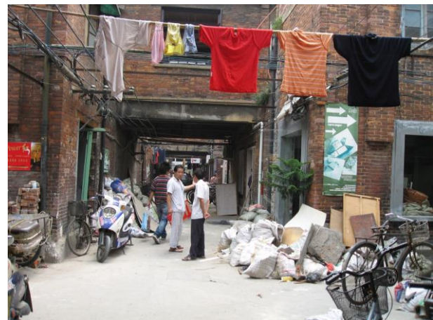
Figure 5b. During renovation (photo by the author)
