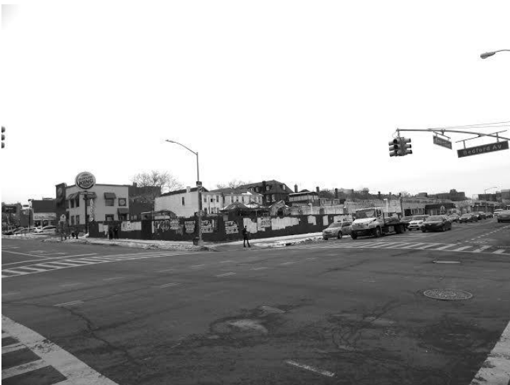
Fig.3 - Construction Site in Area Rezoning for Residential Development, 2015 Photo by Jerome Krase.
