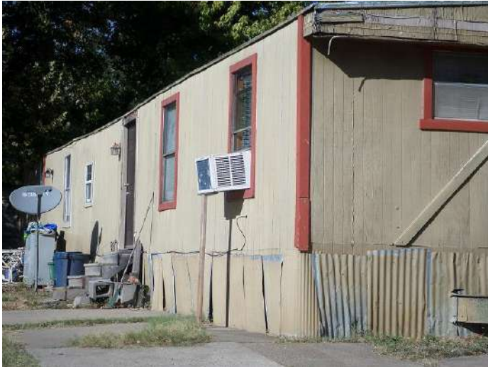
Figure 5. A single-wide trailer in a trailer park in North Texas. Its condition can be described as impoverished and shows clear signs of structural aging and numerous external modifications, including an attached ac window unit. The
