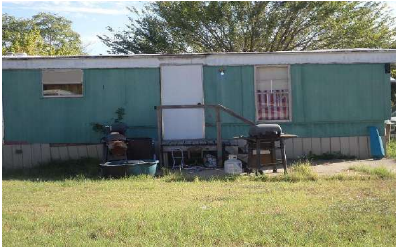
Figure 8. An aging and slowly decaying single-wide trailer. Some of the wooden panelling near the bottom seem to be slightly unbalanced. A wooden stair-case seems to have been added. Paint does not seem to be the original. Numerous appliances are visible near the doorway, including two BBQ grills. The trailer seems to fit into what I characterize as type 2 housing. Photo taken by the author.
